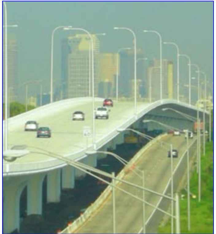
A Tampa expressway authority built three new lanes on six-foot piers in the median strip of an existing tollway. The new lanes, whose cost will be entirely covered by electronic tolls, completely eliminated tollway congestion. Since the new lanes are used inbound in the morning and outbound in the afternoon, the authority likes to say that it built six lanes in six feet of right of way.
