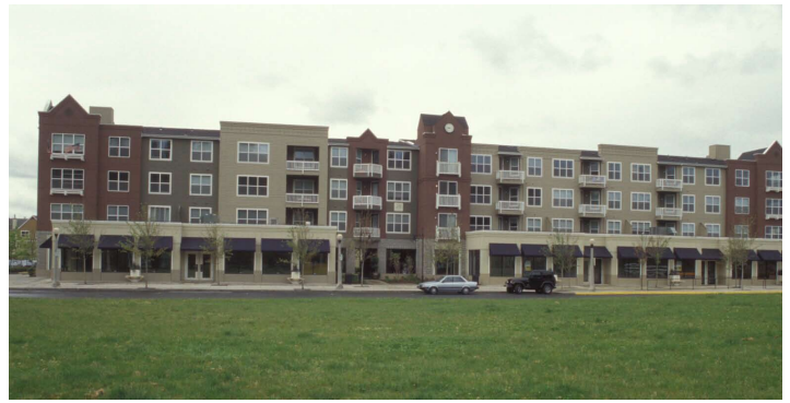
The ground floor of this apartment complex next to Portland's westside light-rail line was supposed to be shops, but after 10 years of vacancies, the owner is turning them into apartments.
